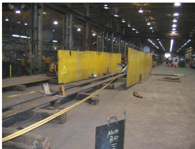
Figure 1 Photo showing the radiographic testing (RT) of a complete joint penetration weld (CJP) with clear area and shielding provided
