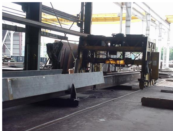
Figure 9 Photo showing the building of girders with their webs horizontal
