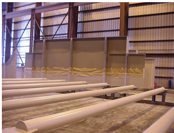
Figure 18 Photo showing painted members in a fabrication shop, note the masked area is for prime coat only
