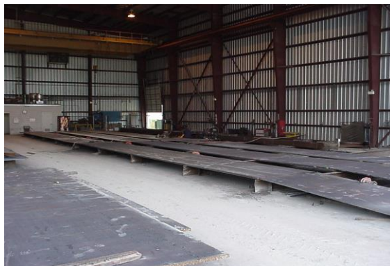
Figure 7 Photo in a fabrication shop showing the butt welding of steel plate slabs
