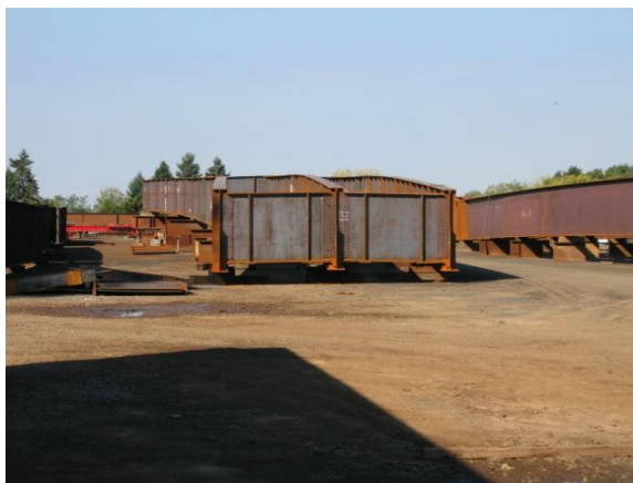
Figure 15 Photo showing the unit assembly of a structure
