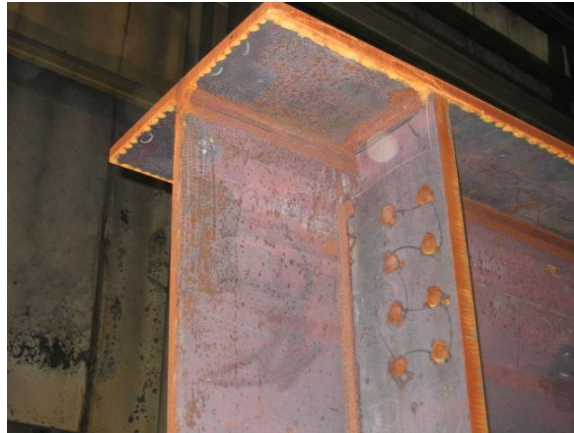
Figure 16 Photo showing a girder before blast cleaning
