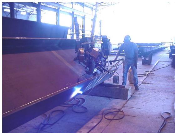
Figure 11 Photo showing the welding of a plate I-girder web to its flange
