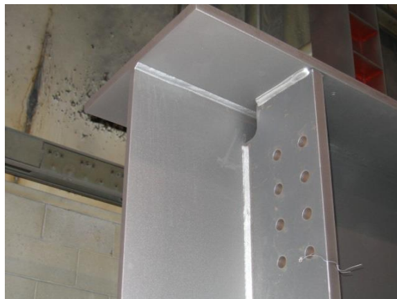
Figure 17 Photo showing a girder after blast cleaning
